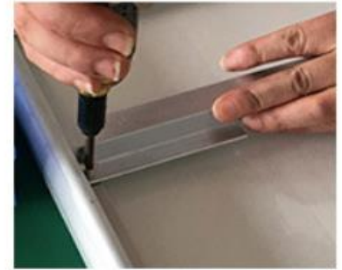
Lamp body beam fixed
